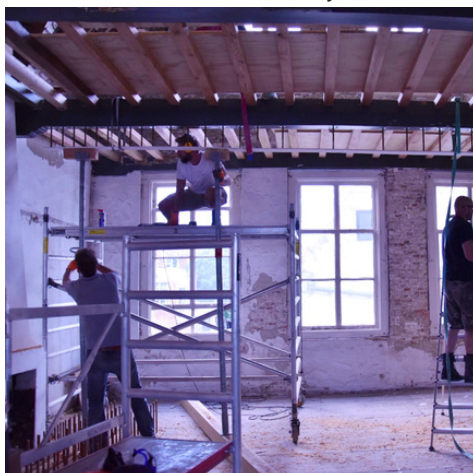
Reinforcing the beams with steel
